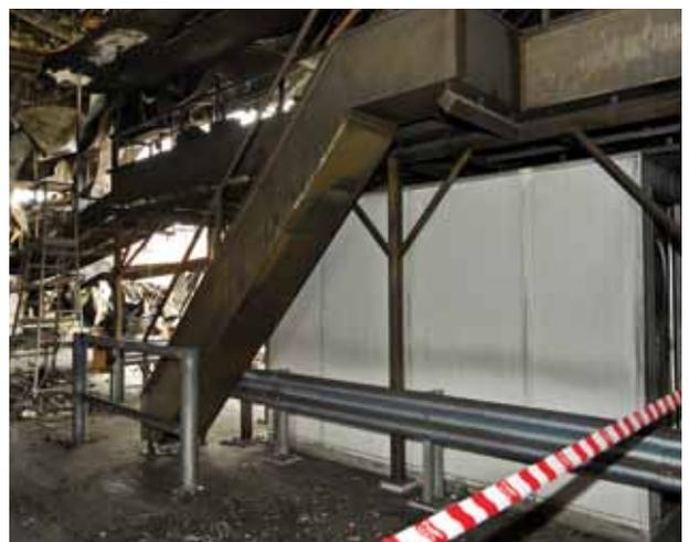
*Kingspan PIR insulated panels remain unscathed after a major fire at a meat processing plant in 2010. Adjacent panels in EPS polystyrene (from another manufacturer) were incinerated.*
