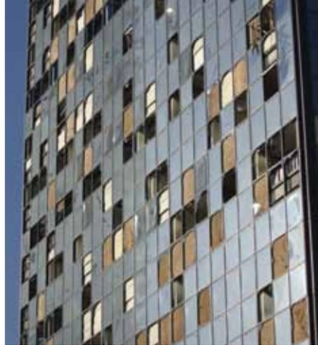
Impact damage can lead to full building cladding failure in severe windstorms.
